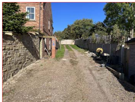
Access Looking up Proposed Driveway
